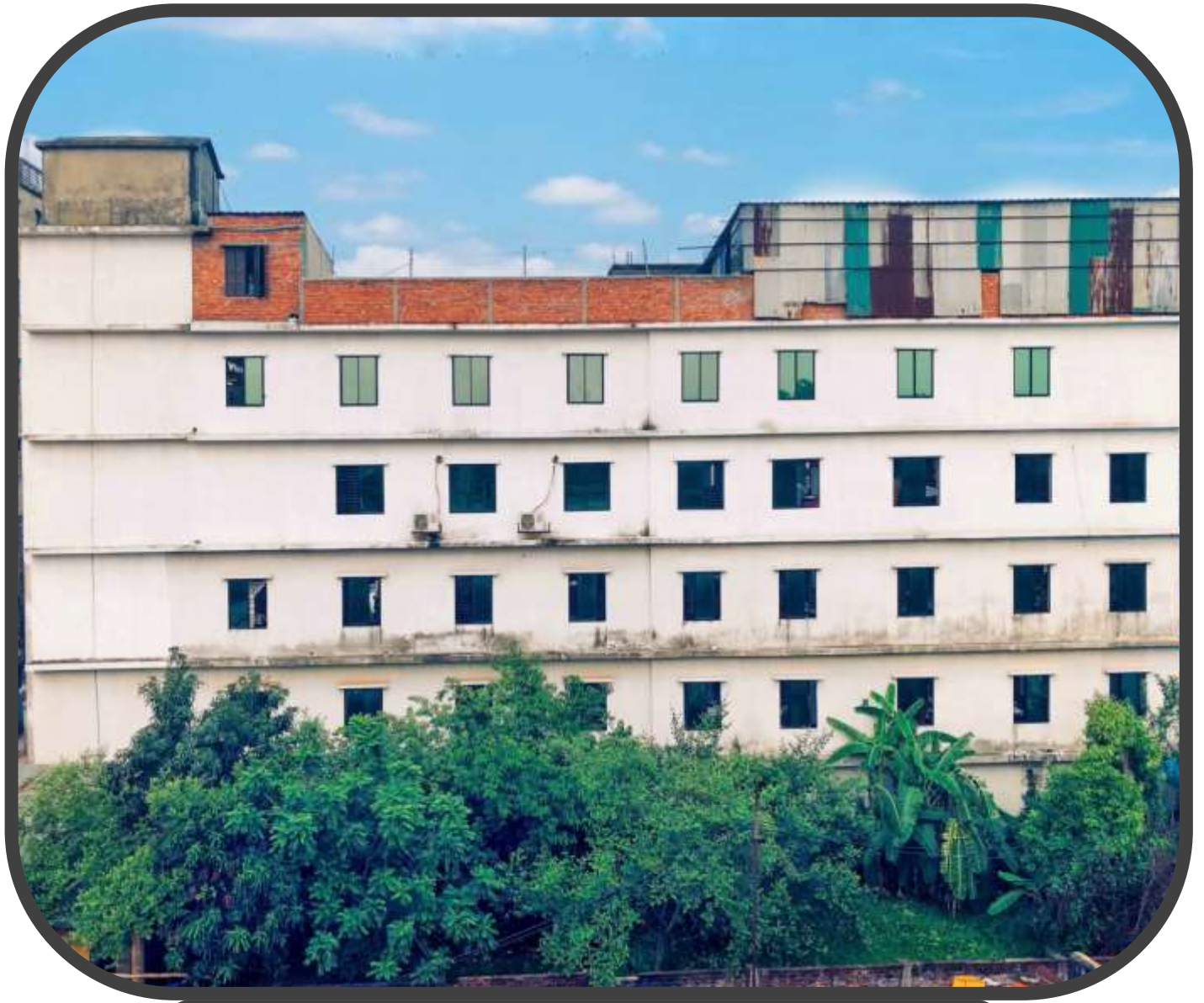
Factory Building (Side view)
