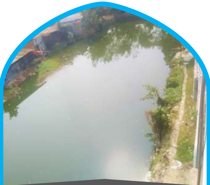
Reserved water for fire safety
